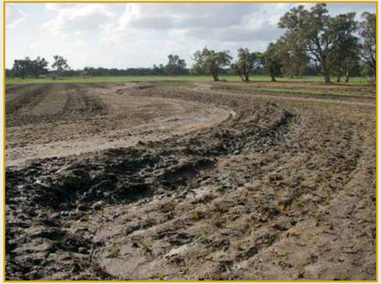
Graded bank construction, May 2011.
