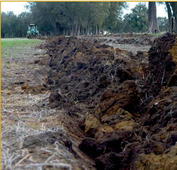
Close-up profile of ripping process.
